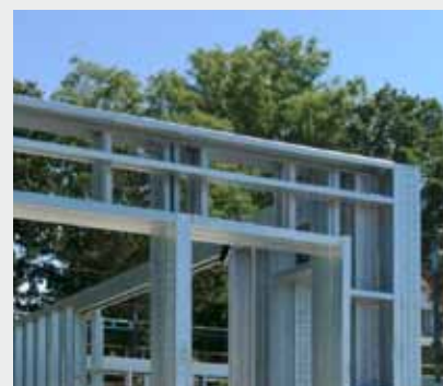
Frame using Lindab's energy beams, ideal for passive houses.
