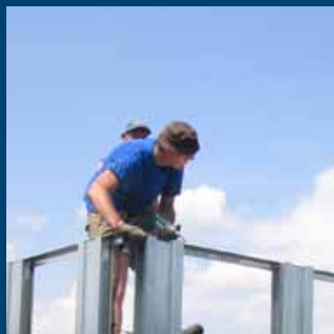
The parts are delivered ready for assembly, minimising the need for welding and cutting on site.
