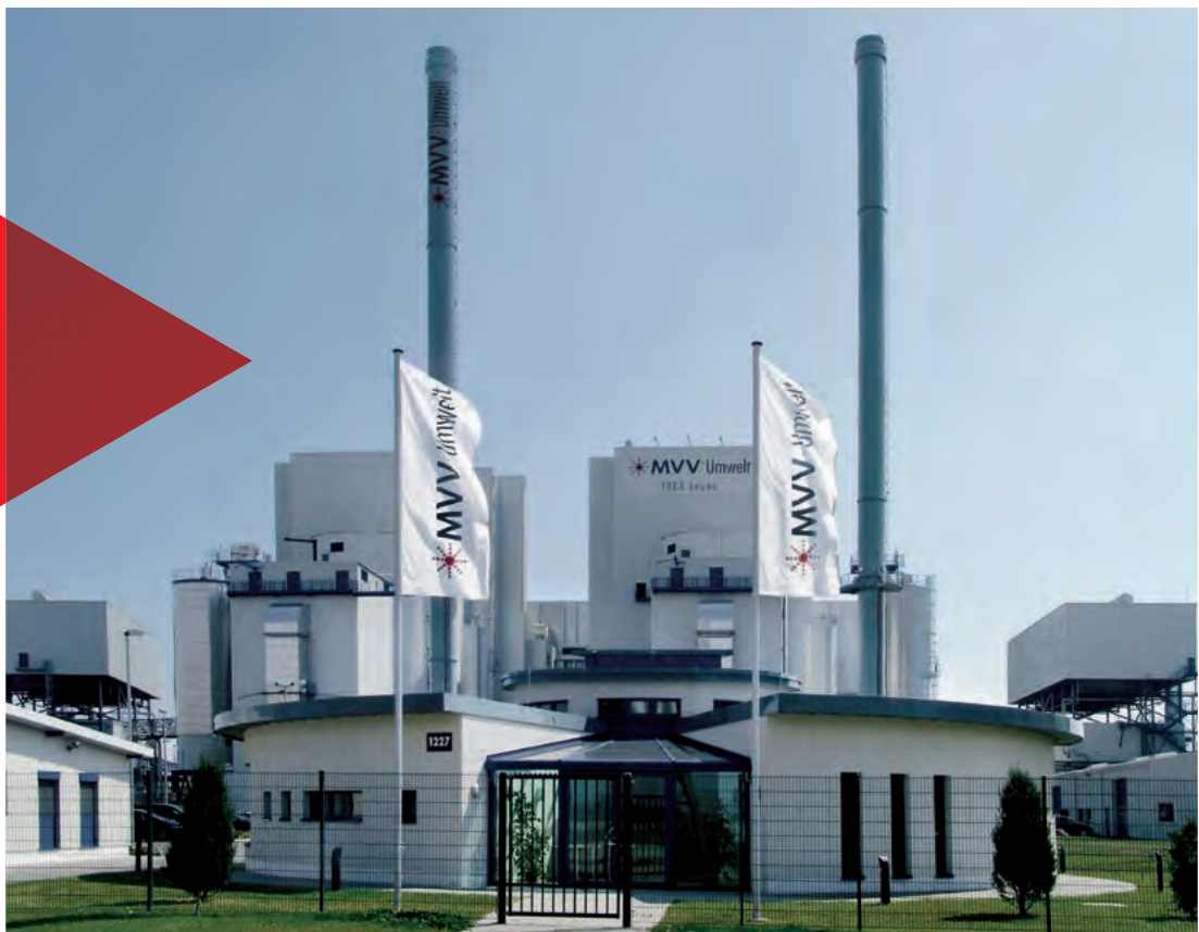
OUR ENERGY FROM WASTE PLANT IN LEUNA
