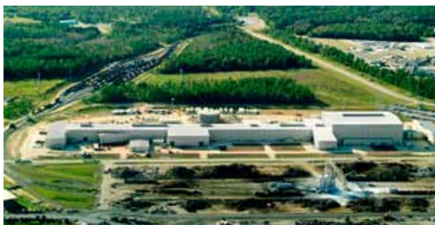
▲ The new quenching line in Mobile.
