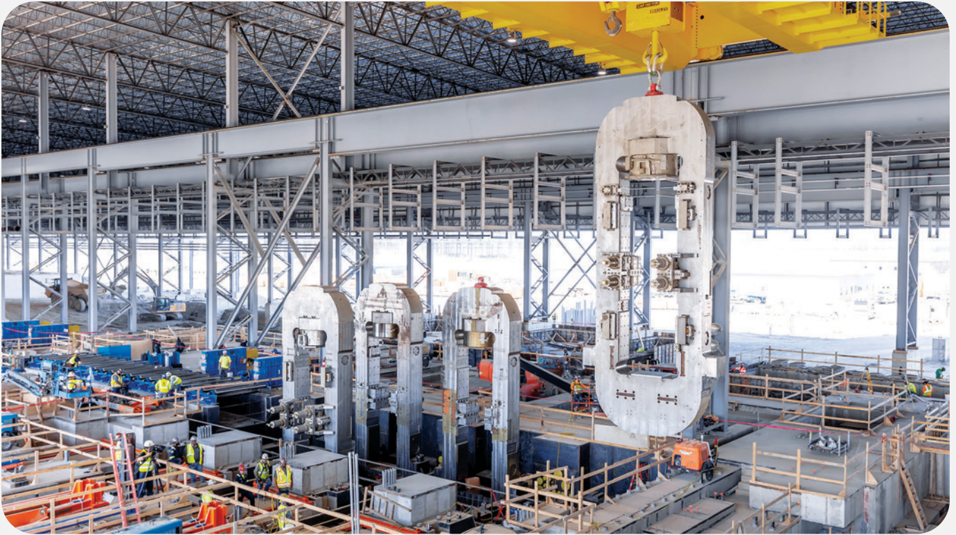
→ Positioning the Mill Stands for the Hot Rolling Mill
