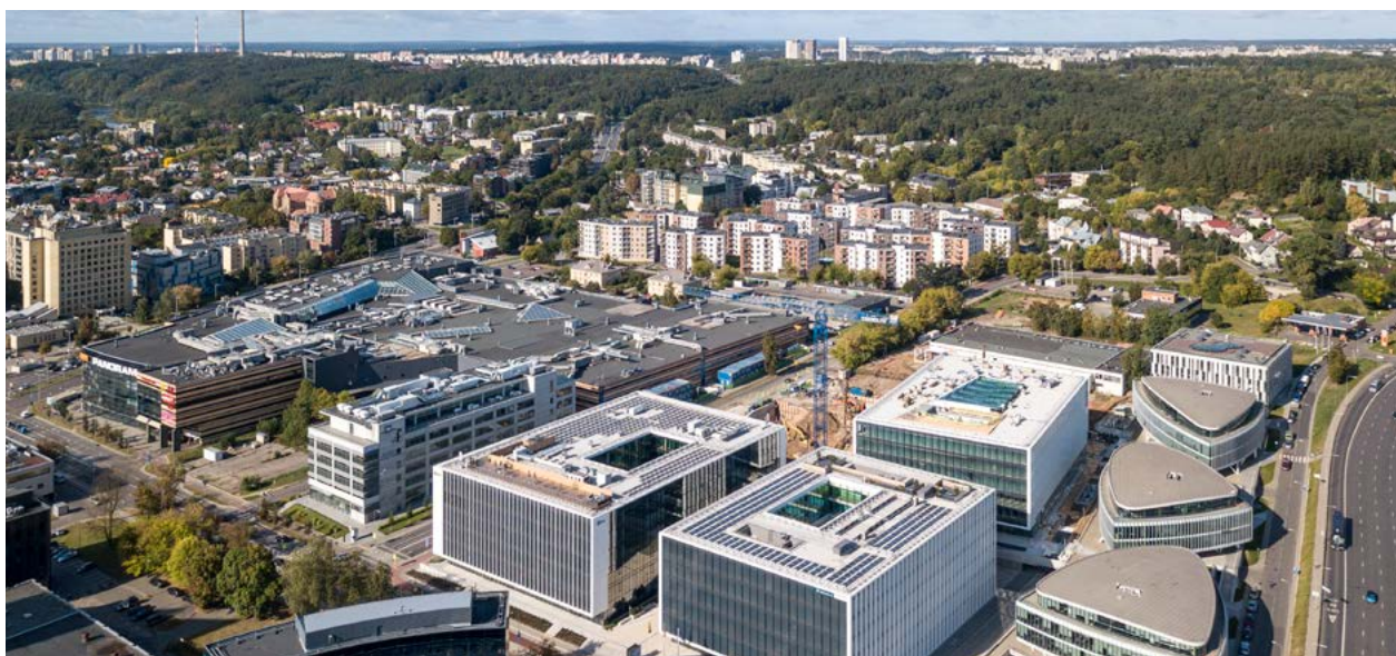
S7-area in Vilnius. S7 (in the foreground), which were acquired by Eastnine in 2019, has solar panels installed on the flat roofs.
