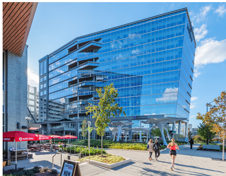
Pictured Above: Vantage South End, Charlotte, NC
