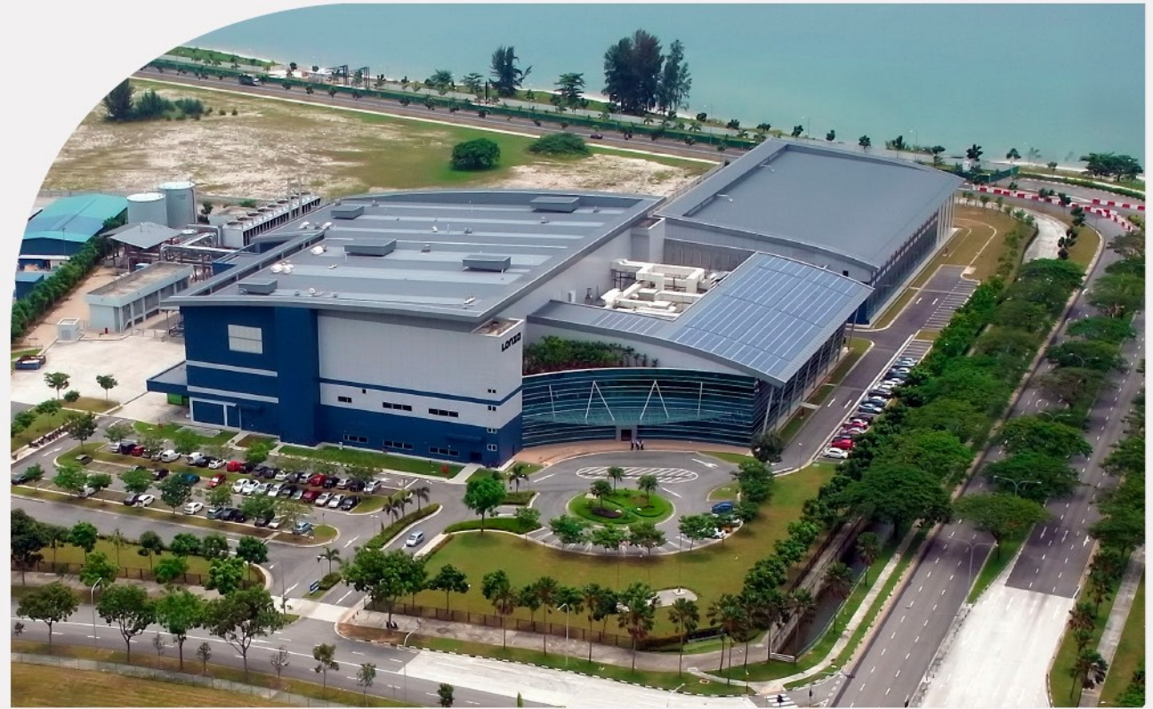
Lonza contract manufacturing facility in Singapore
