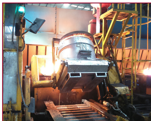
Figure 1: Together, the Ladle Tracker™ and Cast Tracker™ technologies link the core and mould history to the liquid metal history, providing complete traceability.
