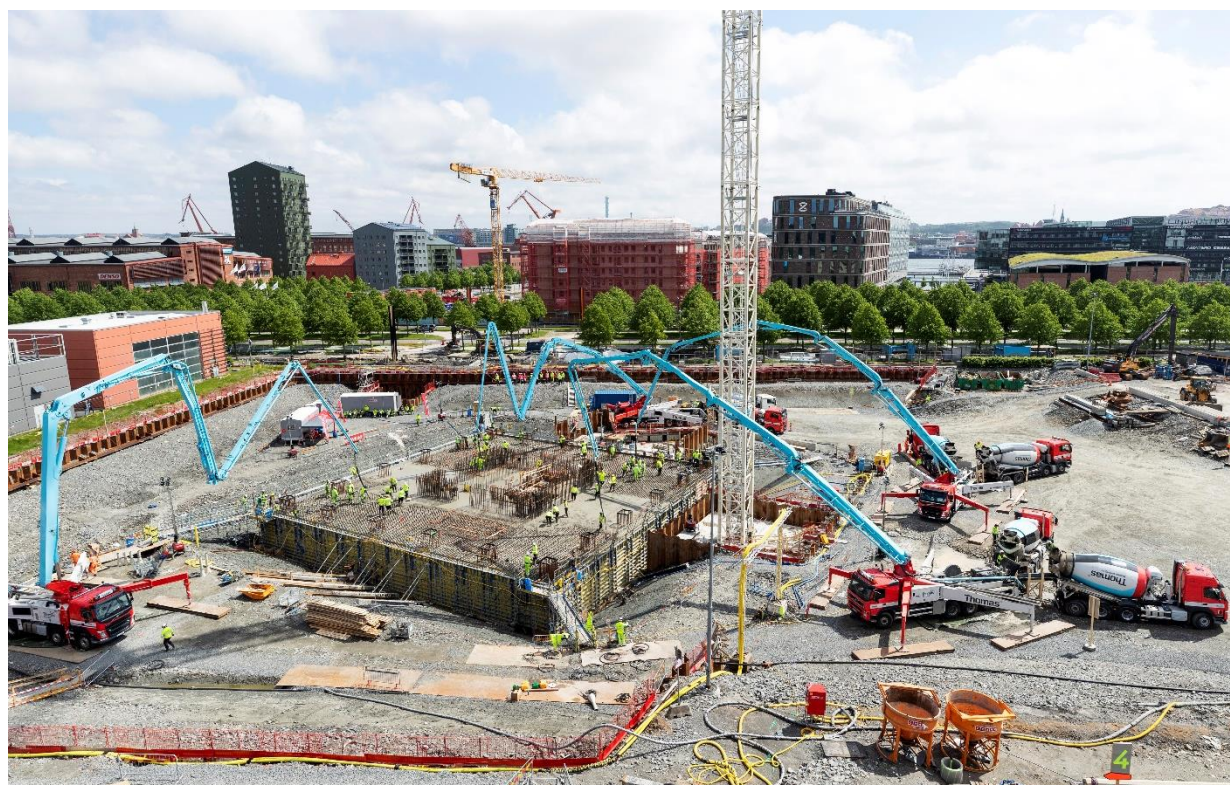
In May, Serneke carried out the casting of Karlatornet's base slab, all in the course of one day.
