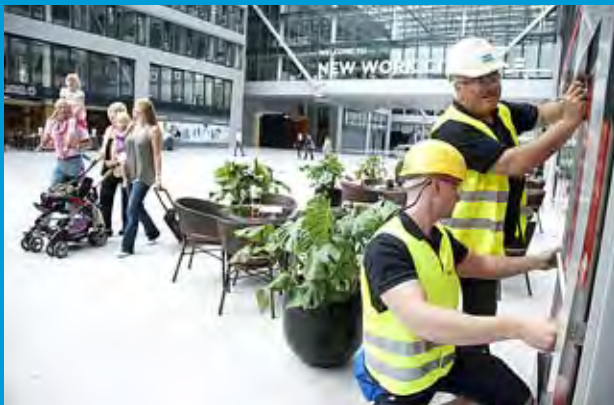
Manfred and Florian are making sure that the fire safety is in order.
