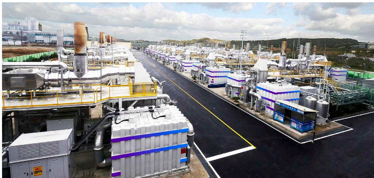
The Hwaseong Baran Industrial Complex fuel cell power platform, which was established in 2013 with FuelCell Energy's design and technology, has the capacity to produce 58.8 megawatts of electricity from 42 fuel cell modules
