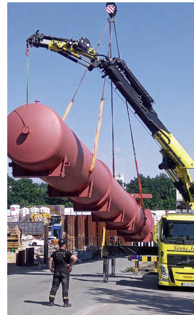
Crane unloading new autoclave in Wittenborn, Germany
