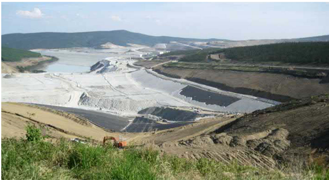
Figure 5: Fort Knox Heap Leach Operation in Fairbanks, Alaska
