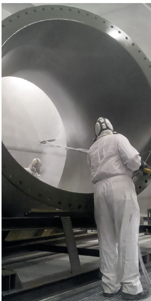
Applying Accoshield corrosion protection coating
