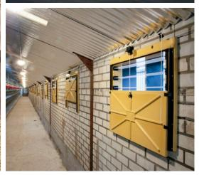
TPI Polytechniek's OmniFlux inlets installed in Dutch poultry farm
