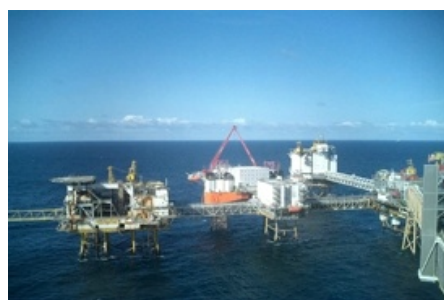
HVAC facility for ConocoPhillips
