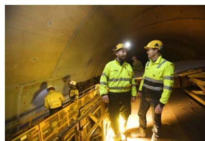
Construction work on railway tunnel to Tønsberg
