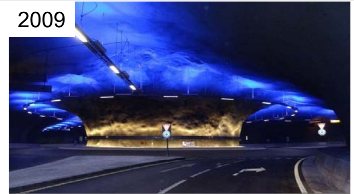
T-Connection, NOK 878 m
