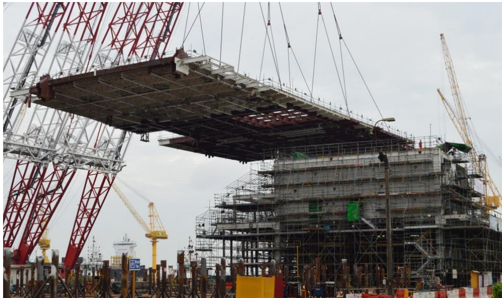
The 3 500 m2 intermediate deck fit well together with the cellar deck
