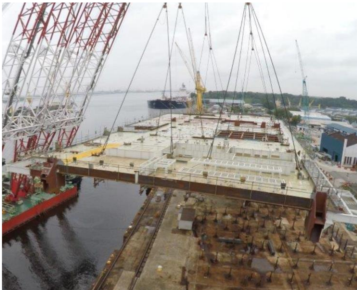
30 January 2015: Lifting of the intermediate deck
