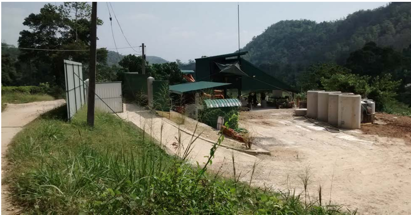
Shaft H site development area
