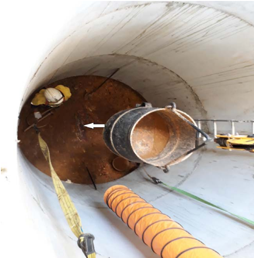
Shaft J 2.5 metres liner showing weathered graphite vein in shaft
