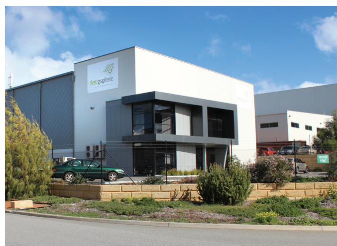
100 tonne/year manufacturing facility at Henderson, WA
