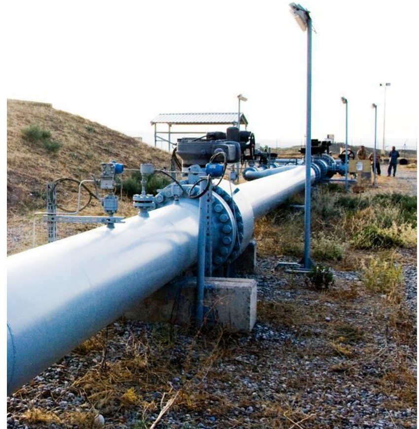
Fishkabour pipeline tie-in point.
