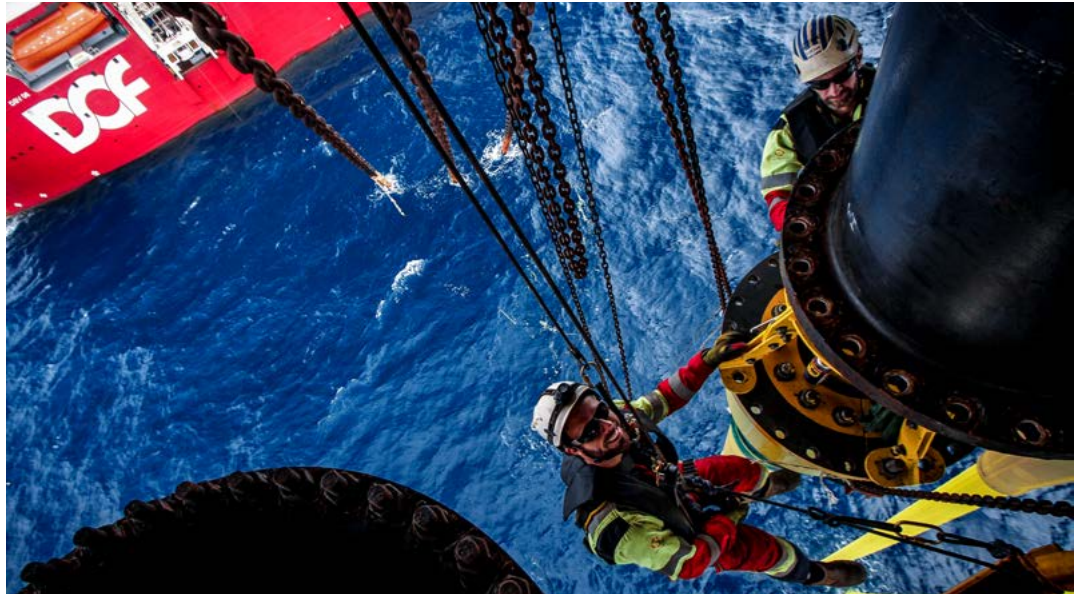
Two Subsea engineers working with an FPSO hookcup
