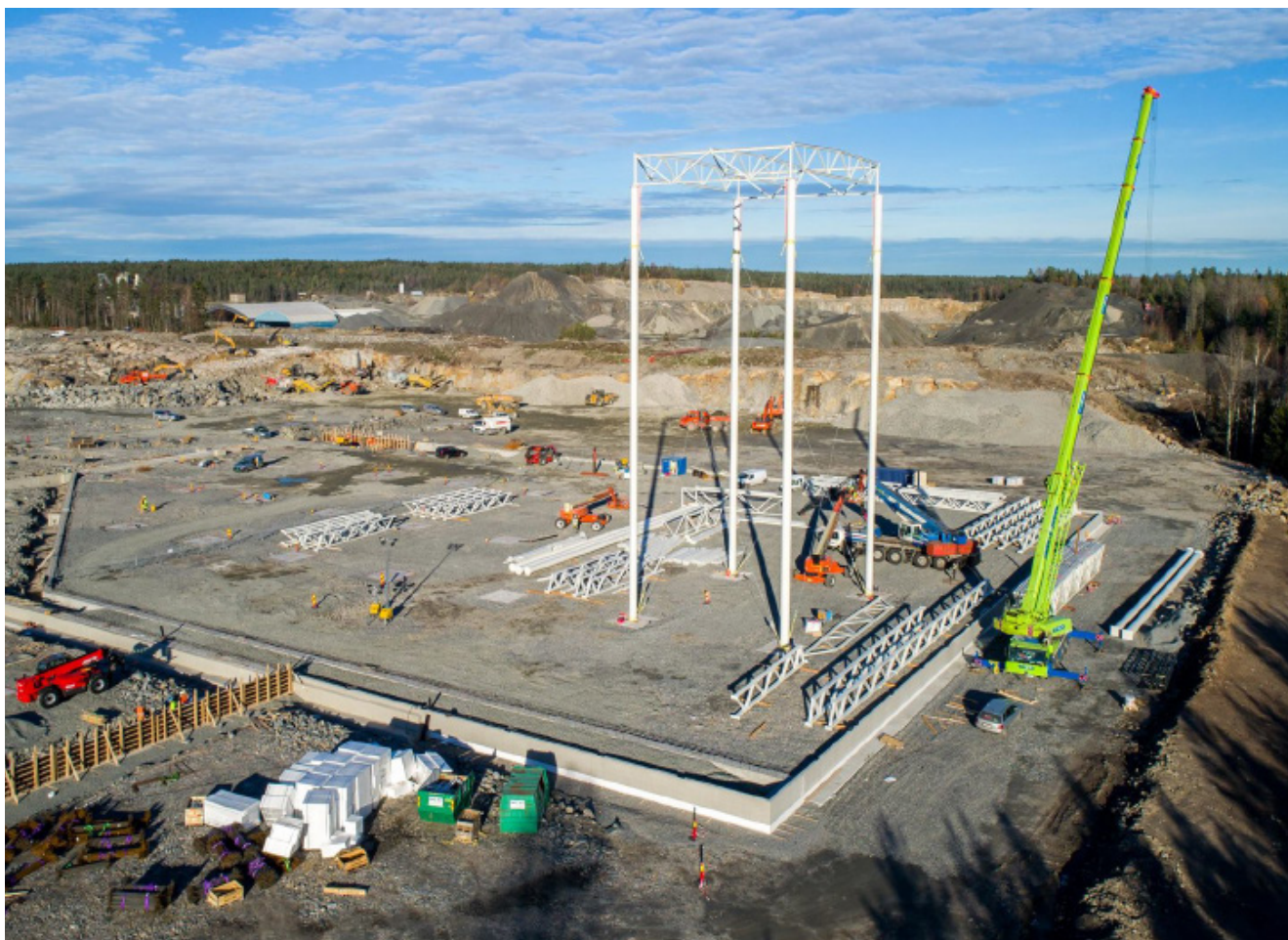
New central warehouse progressing as planned
