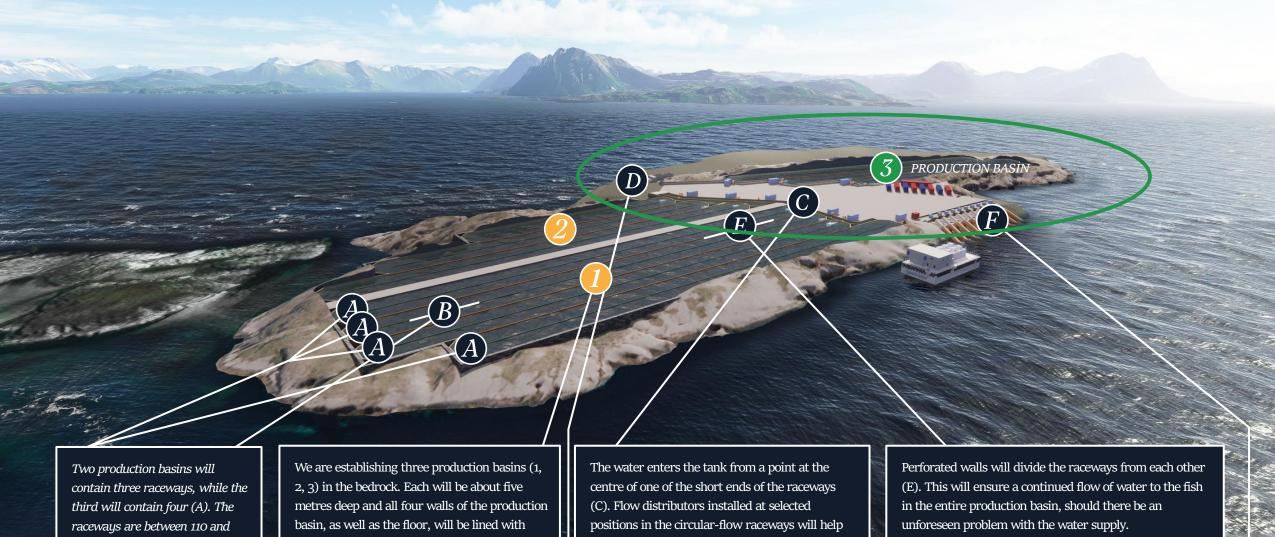
214 meters long and are fitted with a dividing wall (B) in the centre, which facilitates the circulation of water.
