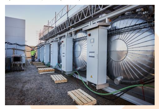
The Heatcube represents an innovative, low-cost and modular solution for thermal energy storage and can use multiple renewable energy sources to heat molten salt to over 500 degrees Celsius. The high-temperature salt is then used to produce steam or a combination of electricity and hot water for industrial use and as input to district heating systems.
