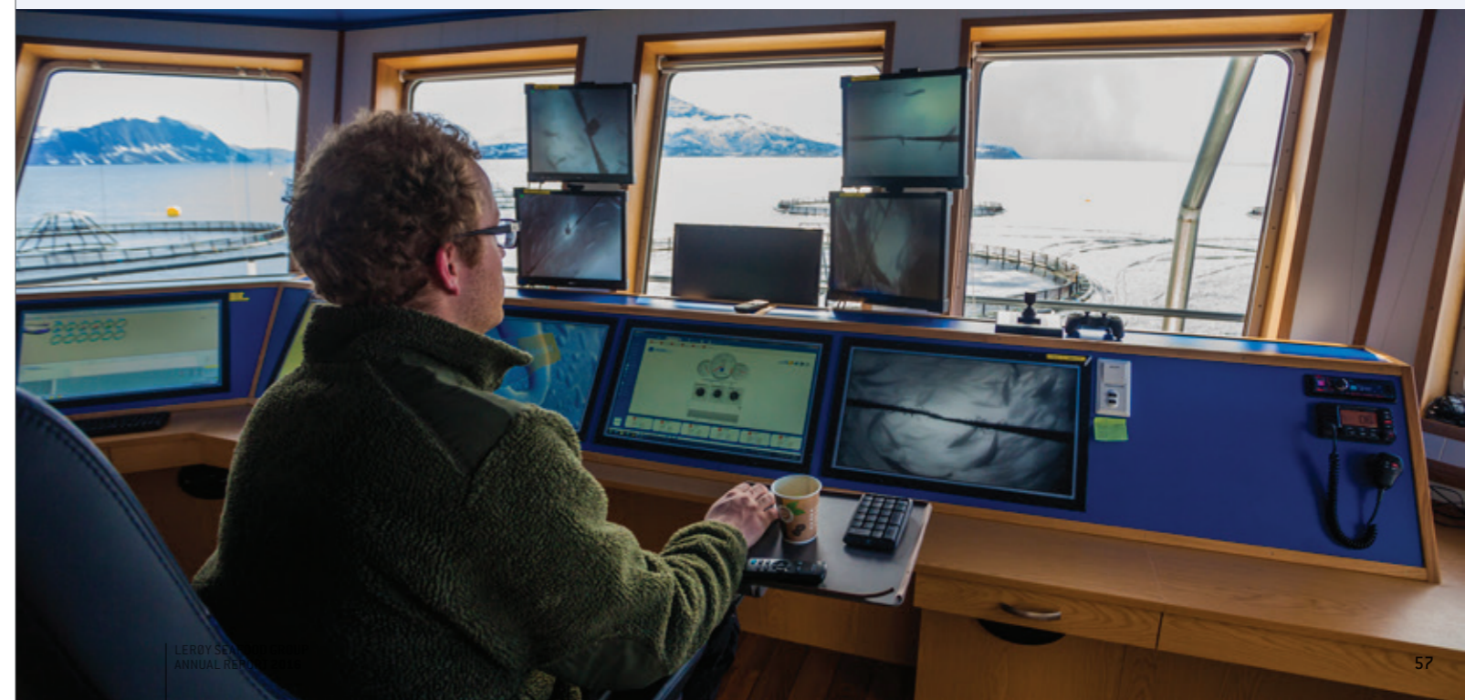
The control room on the barge
