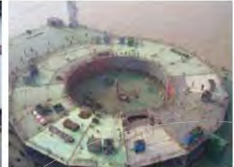
Submersible construction barge/a float
