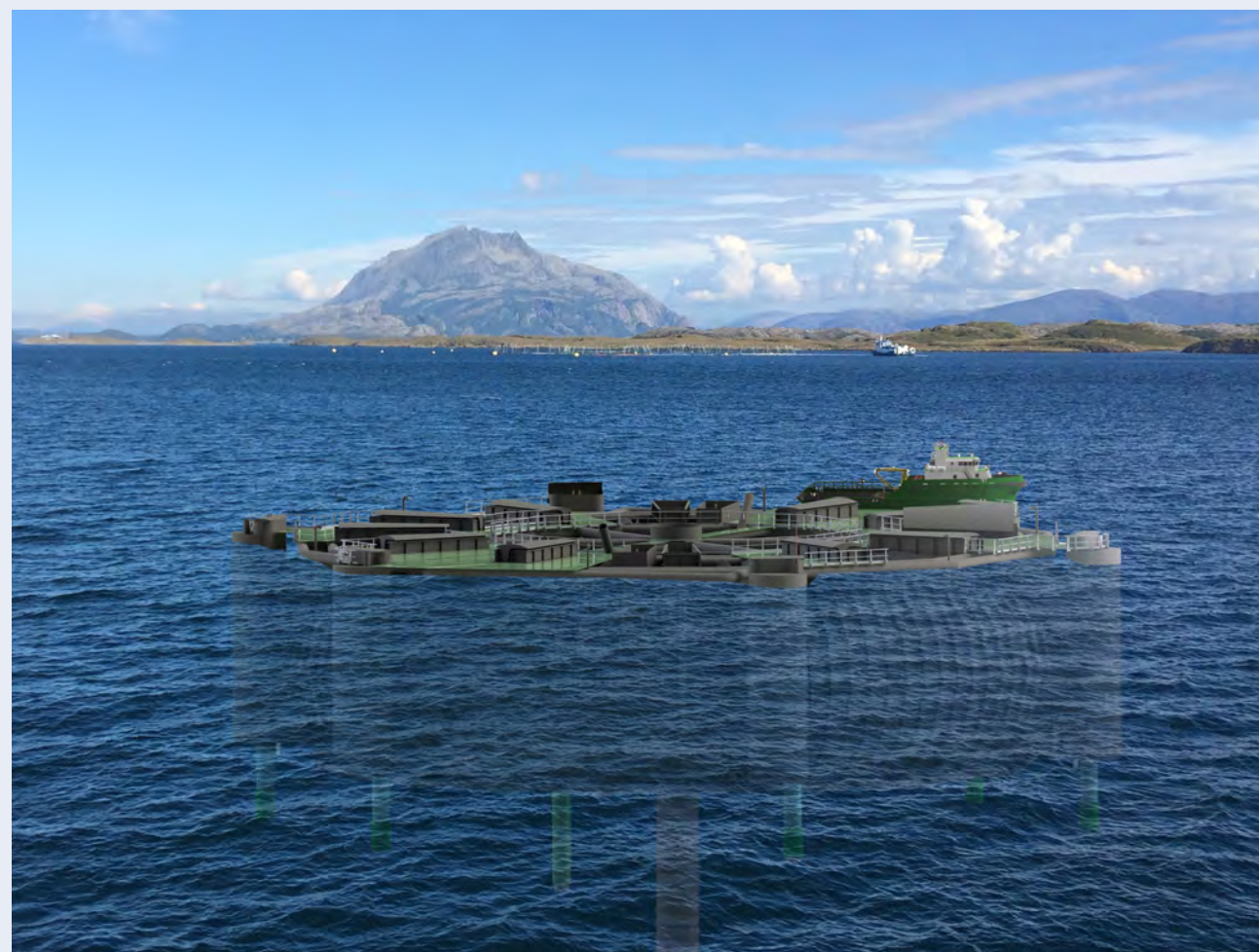
The Marine Donut is 3 000 m3 with high circulation.
