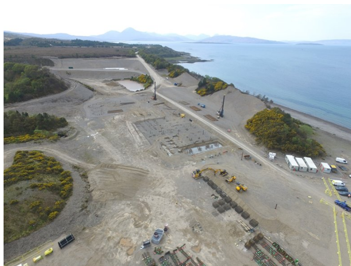
Construction of the feed plant at Kyleakin has started. At this stage, the primary activity is piling.
