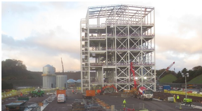
Construction of the feed plant at Kyleakin.
