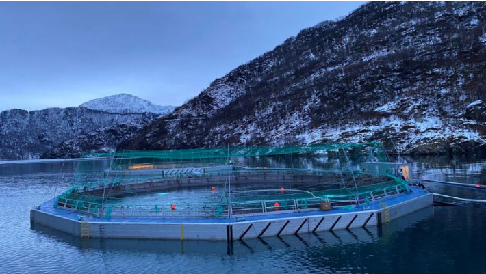
Norway - Closed Containment System
