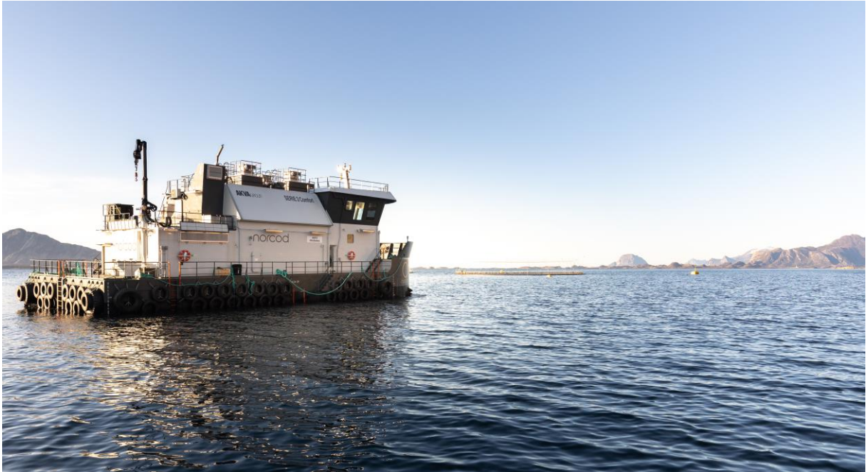
The electric feed barge at Norcod's Frosvika facility now using power from shore (Photo: Norcod)
