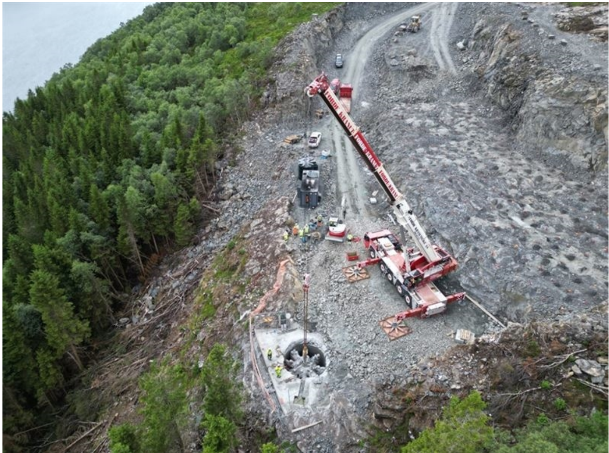
Picture 1. Final lifting out the drill from the ore pass before securing
