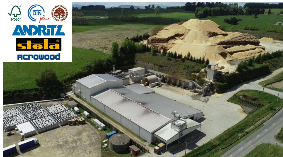
Nature's Flame modern and state-of-the-art wood pellet production facility in Taupo, New Zealand
