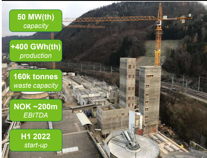
Waste-to-energy plant being installed in Bruck, Austria
