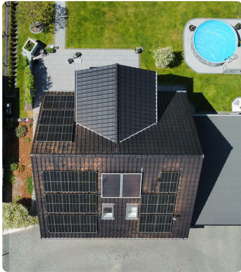
Otovo installation in Brandenburg, Germany. Q2 2022
