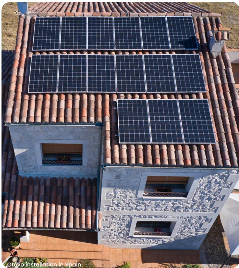
Otovo installation in Spain
