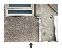
There are various types of cladding, here we can see a building clad with combustible insulation, with concrete render over
