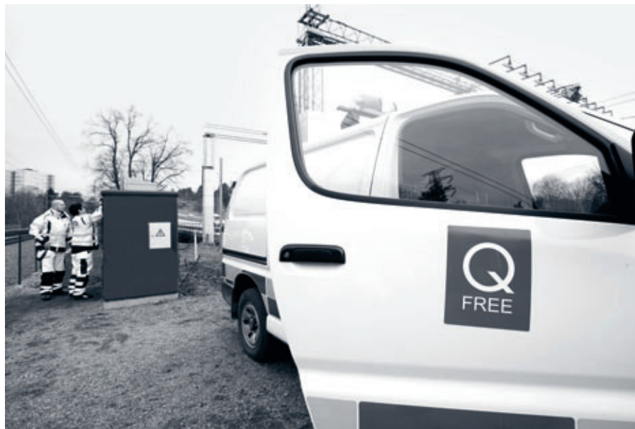
SERVICE AND MAINTENANCE ON SITE >
