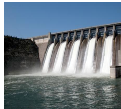
Shafts for water turbines
