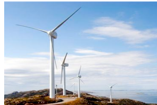
Main shafts, gearboxes, generator shafts and integrals
