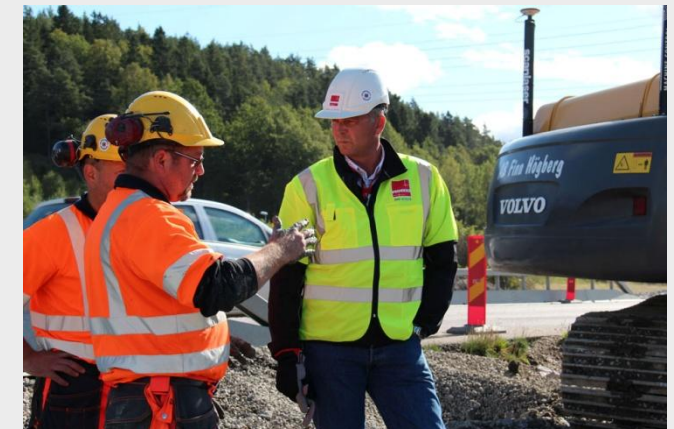
Work is well underway at the E45, south-west of Trollhättan in Sweden
