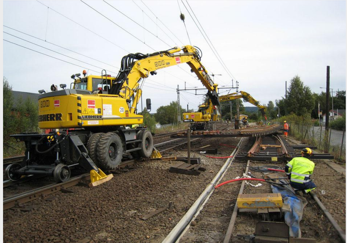
Maintenance of rail network
