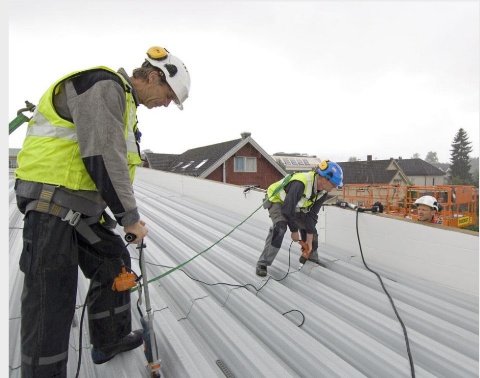
Roofing on a new building for Rema 1000 in Hokksund
