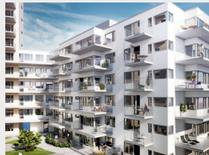
Brf. Resdens Sannegården, Gothenburg
