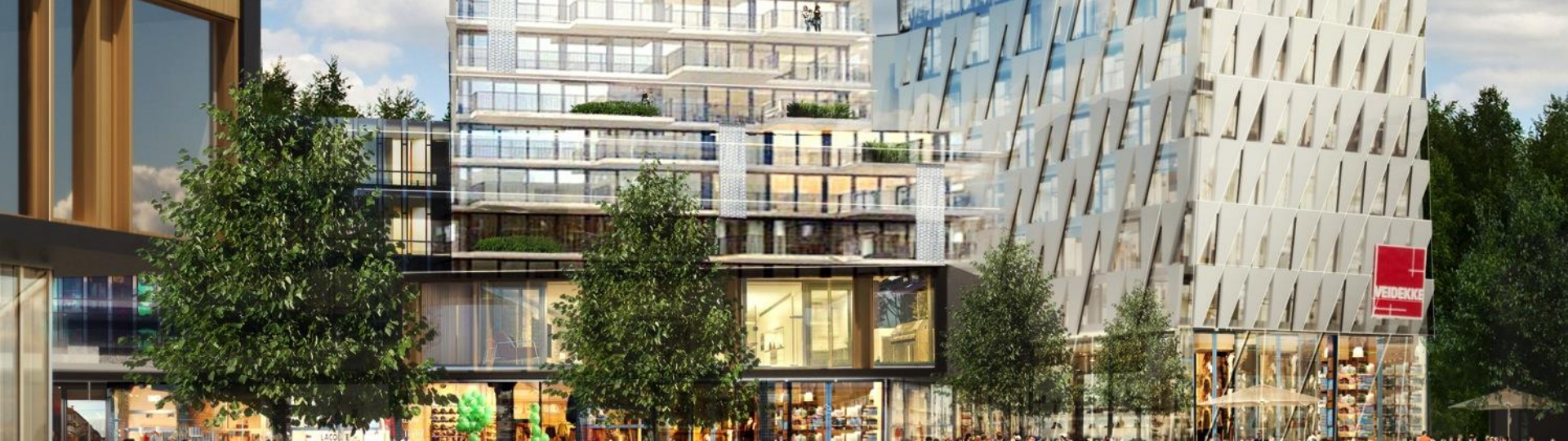
Veidekke's new HQ in Skøyen
