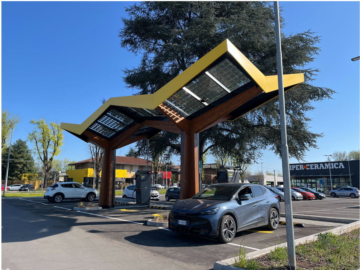
Fastned's charging station in Castellanza, Italy opened in March 2026.
