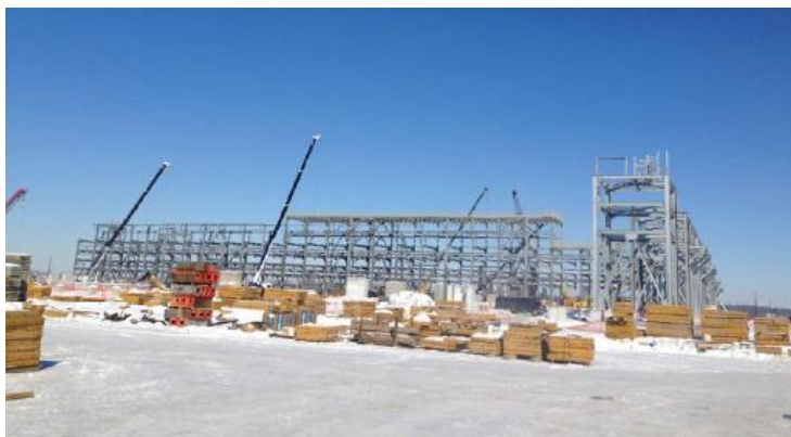
Ammonia steel structure erection
