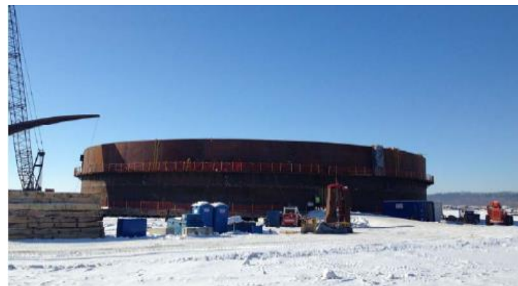
Ammonia tanks shell rings installation
