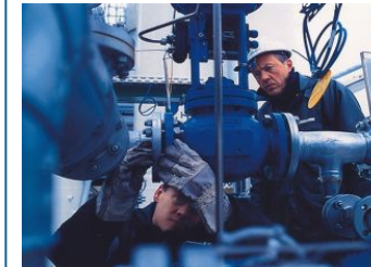
Flange sealed by a gasket
