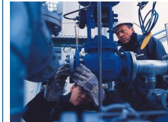
Flange sealed by a gasket
