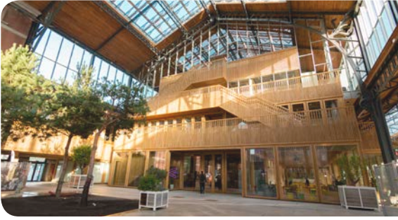
Extensa - Tour &amp; Taxis - Gare Maritime - Brussels
