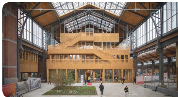
CFE Contracting - Gare Maritime - Brussels
