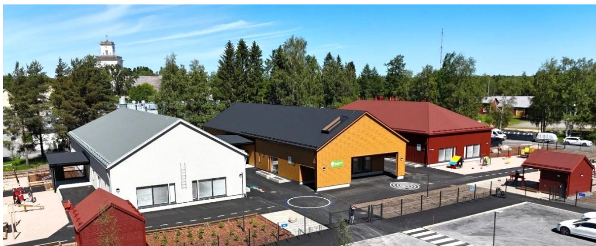
Kokkola Kruunupyöntie in Kokkola (Finland) Child day-care centre completed in July 2025
