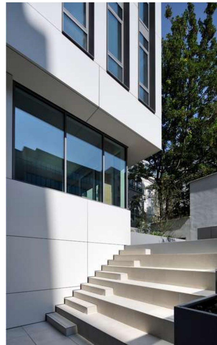
► Office building Montoyer 10 (M10) – Brussels' CBD (BE)
