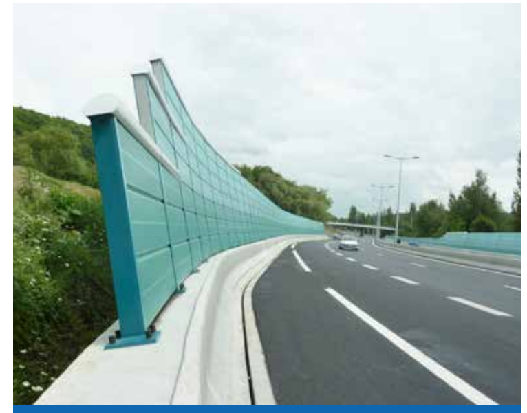
Cyclefoam sound wall in Le Havre, Rocade Nord
