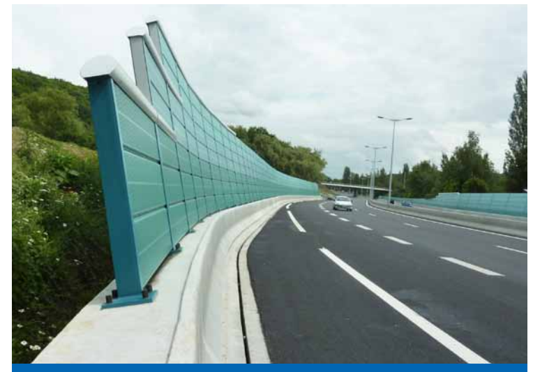
Cyclefoam geluidswand in Le Havre, Rocade Nord
